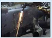
**A WARNING** Be careful not to not damage the frame rail. Only torch the head of the bolt.
