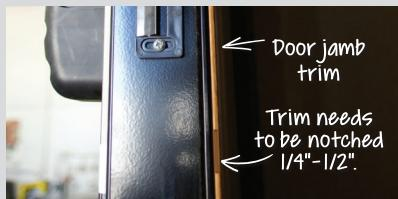
If there is trim on the back side of the door jamb that protrudes, it will interfere with the latch on the step. The trim will need to be notched 1/4" - 1/2" to accommodate the latch.
