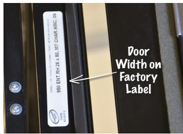
If there is no label, then on the inside of the door frame, measure from flange to flange at the base of the door. Refer to the Fit Chart on the last page for the door width. Keep in mind that the flange-to-flange measurement needed is the narrowest part of the entry door.
